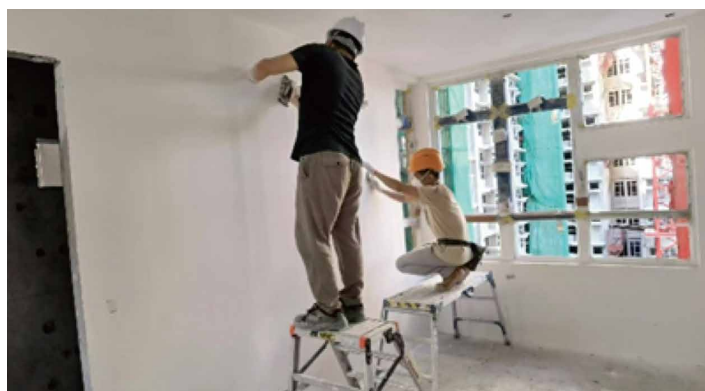
Final touch-up by workers after robot completed the coating work
