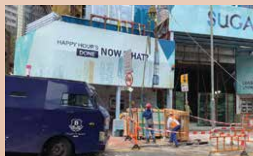
Figure 1) Construction work in the roadside
