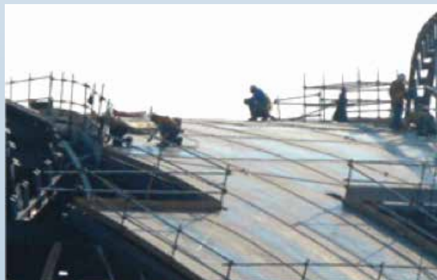
Figure 4) Prefabrication of Roof Structures at Hong Kong International Airport
