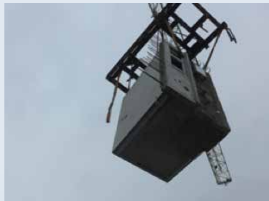
Figure 3) Lifting of Precast Bathroom
